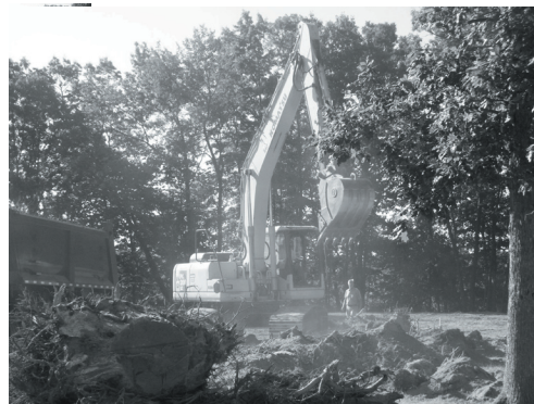
Dale Cook (1981) of Cook Brother's Excavating removing stumps for the new ball field as Keith Cook (1973) looks on.
