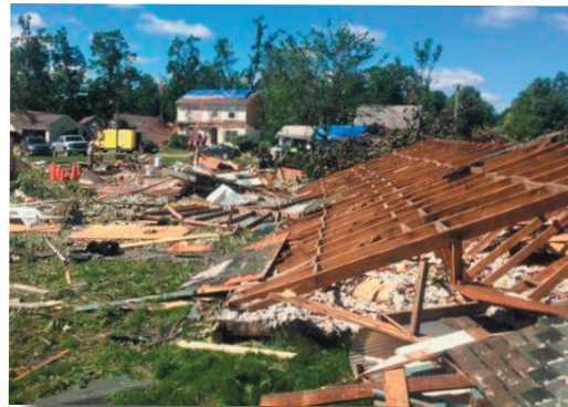
The remnants of the pole barn on Father Flohe Field after the tornado.
