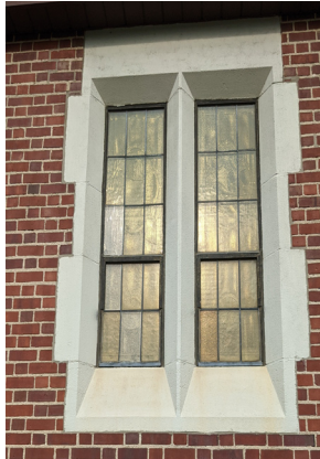
Clear safety glass now covers the stained glass windows in the Chapel (left) in place of the amber colored glass that covers the stained glass windows in the body of the church. The clear glass protects the windows from damage and also lets the stained glass designs show through when the church is lighted at night.
