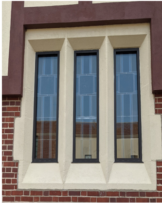
Clear safety glass now covers the stained glass windows in the Chapel (left) in place of the amber colored glass that covers the stained glass windows in the body of the church. The clear glass protects the windows from damage and also lets the stained glass designs show through when the church is lighted at night.
