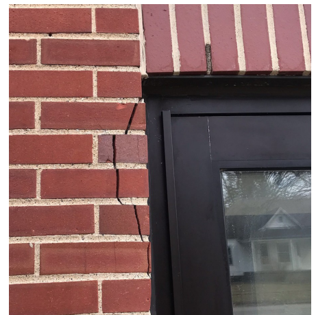
Cracks in the bricks and missing mortar in the joints need immediate attention.
